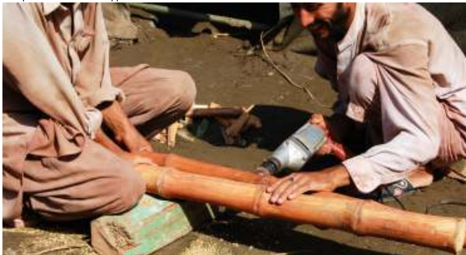
Artisan trainees prefabricate beams and joists
