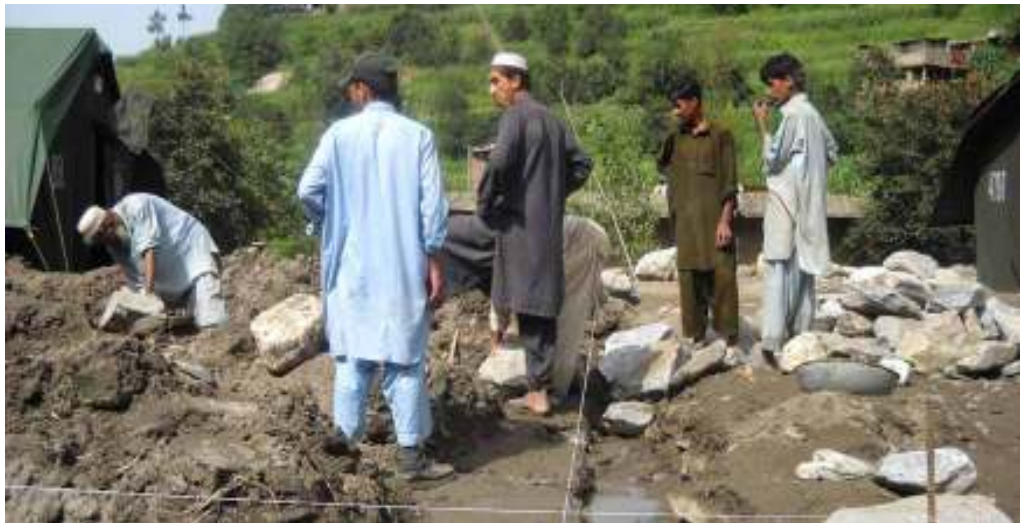
Community member assist in excavation of foundations and laying pad
