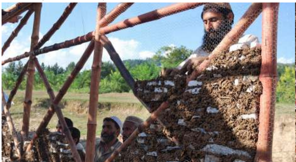
Artisans Work on Dhijji infill with Stone
