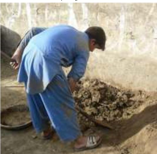
Community members prepare mud lime mixes for mortar
