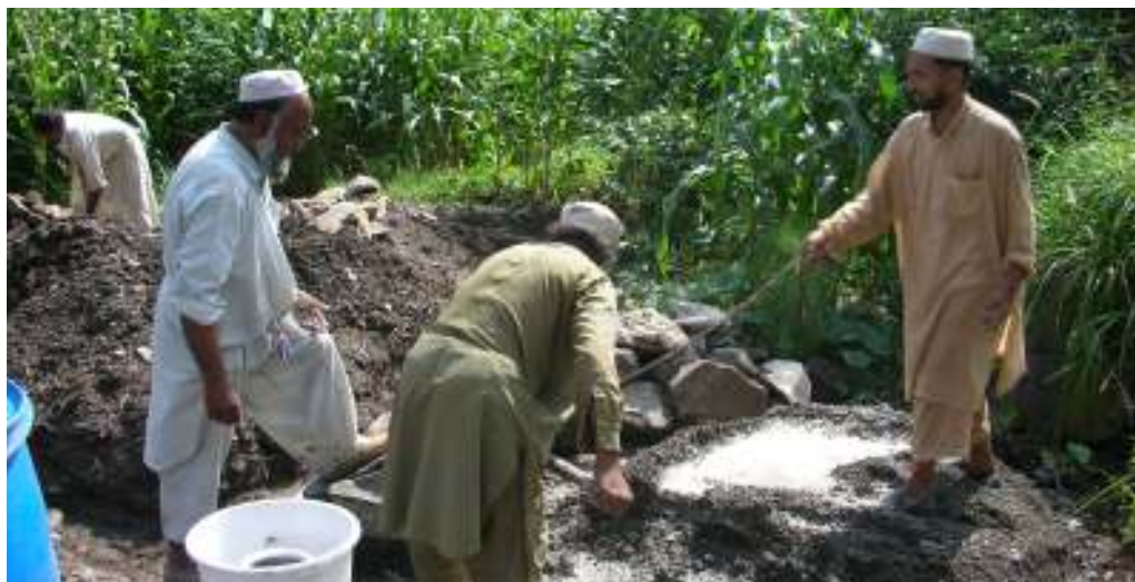
Household members mixing ortar and dressing stone for foundations
