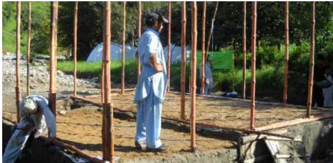
HF skilled artisans erect bamboo posts
