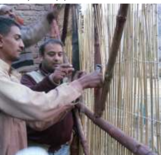
HF team teaches local members how to secure bamboo matting to structure
