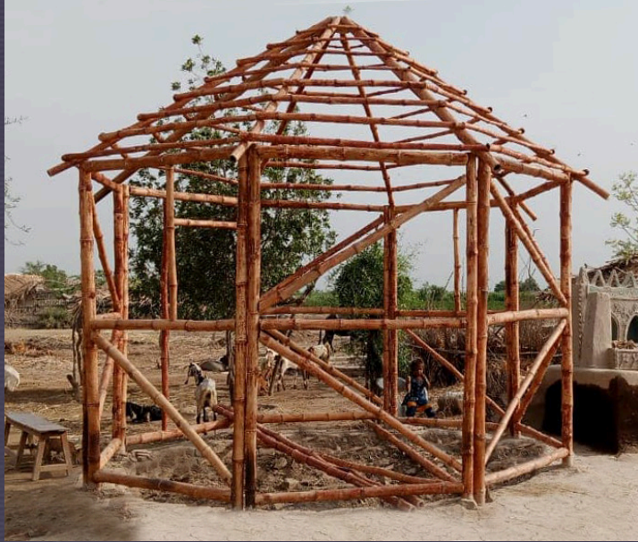
1. Prefab Bamboo Skeleton erected in 2 hours.
