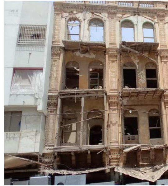
Demolished from inside. Waiting for facade to collapse.
