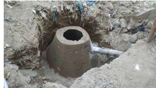
New manholes by Sewerage Board.
