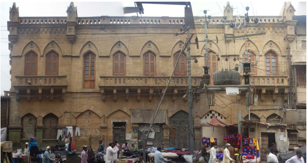
Before intervention. Denso Hall facade marred due to misuse and attachment of electrical equipment,
