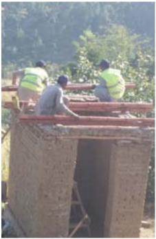
Learning about bamboo jointing and placing bamboo joists on roof.
