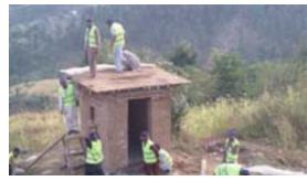
Completing the roof for receiving water proof layer of lime pozzolana.
