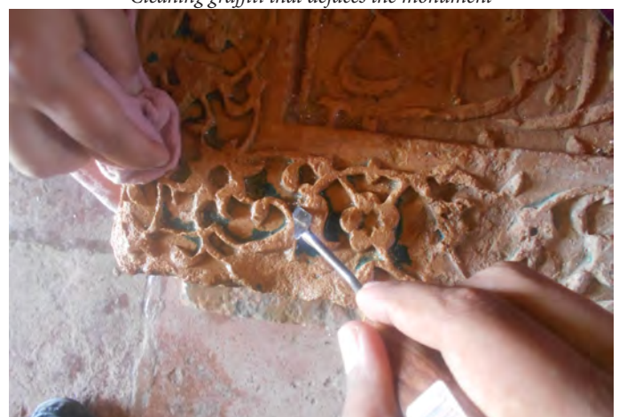
Removing tough enamel paint from groves between stone carving
