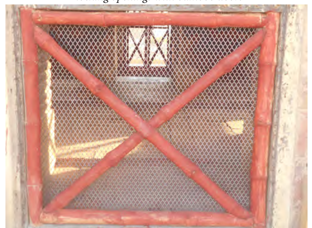
Placement of metallic mesh on all openings
