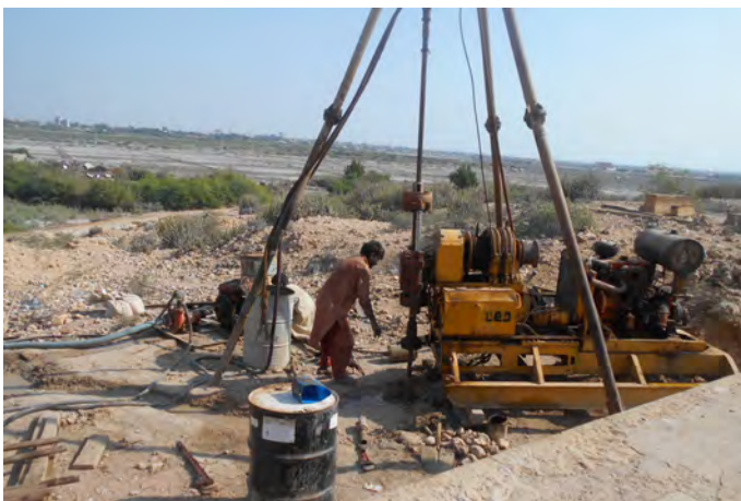
Setting up of the second, much larger machine for soil investigation
