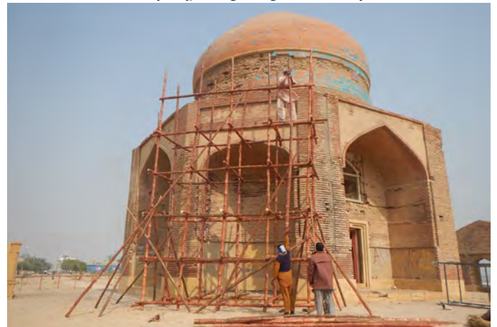
Erection of Bamboo Scaffolding along South-West Facade
