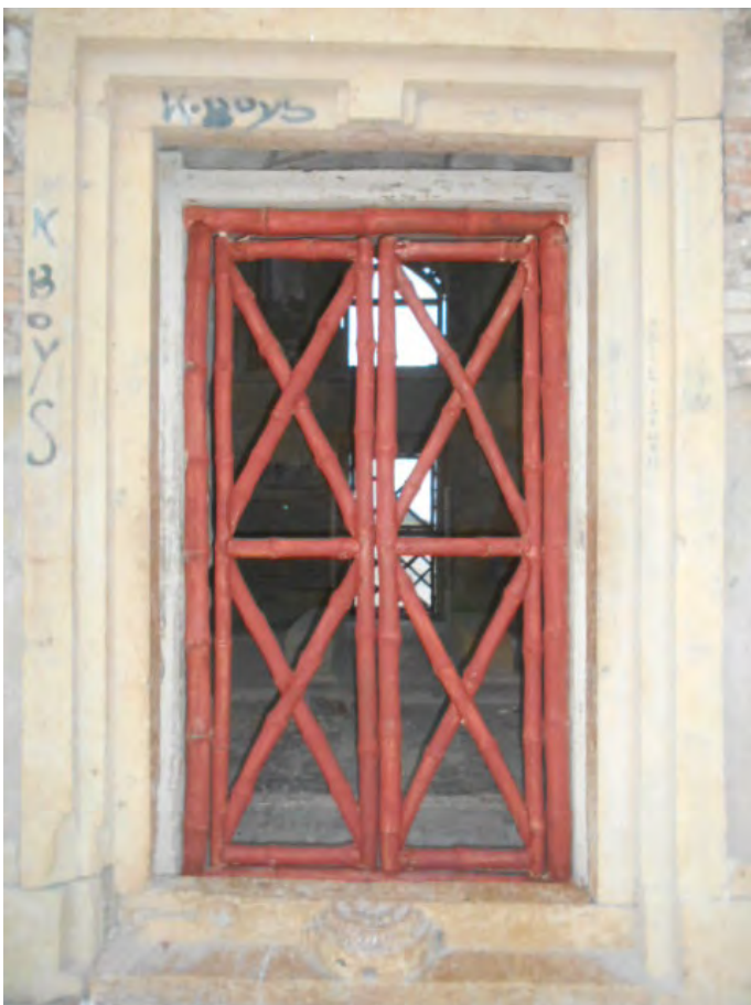
Blocked opening with bamboo door
