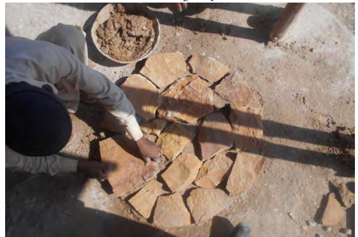
Stone flooring being prepared on Site
