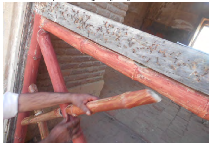
Blocking openings with bamboo doors
