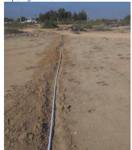
Installation of water supply line at Makli
