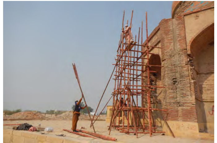
Erection of scaffolding along South-West facade
