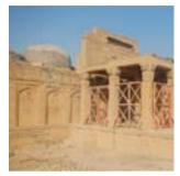
The stone tomb of Jan Baba, originally an enclosure, that later seems to have acquired entrance and grave canopies along iwith separation of a zenana enclosure. The graves canopy has suffered due to the settlement in the middle chamber and loss of two valuable domes. The effort is to maintain the original stone work as well as preventing the collapse of the middle dome fabricated with neatly arraigned carved stone tiles. The project is supported by the German Government.
