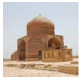
The imposing brick tomb of Sultan Ibrahim and the stone enclosure tomb of Amir Sultan are being conserved with support fom US Ambassador's Fund for Cutural Preservation. The work requires careful handling due to the fragile state of masonry and glazed tile (kashi) work, much of which has been lost due to neglect and pilferage. While conservation of the masonry is progressing, kashi work will be undertaken once the UNESCO Project for Revitalization of Ancient Tiles finalzes its recommendations.
