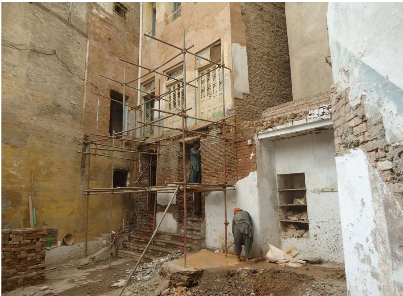
During demolition of Non-historic front portion.
