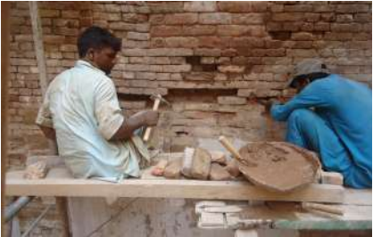
Underpinning brick masonry
