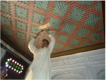
Replacing damaged tarseem bandi.
