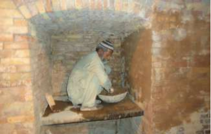
Re-pointing mortar joints in niches.
