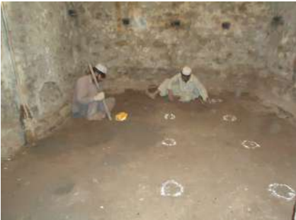
Marks made for boreholes in the basement.
