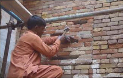
Filling missing bricks and re-pointing.
