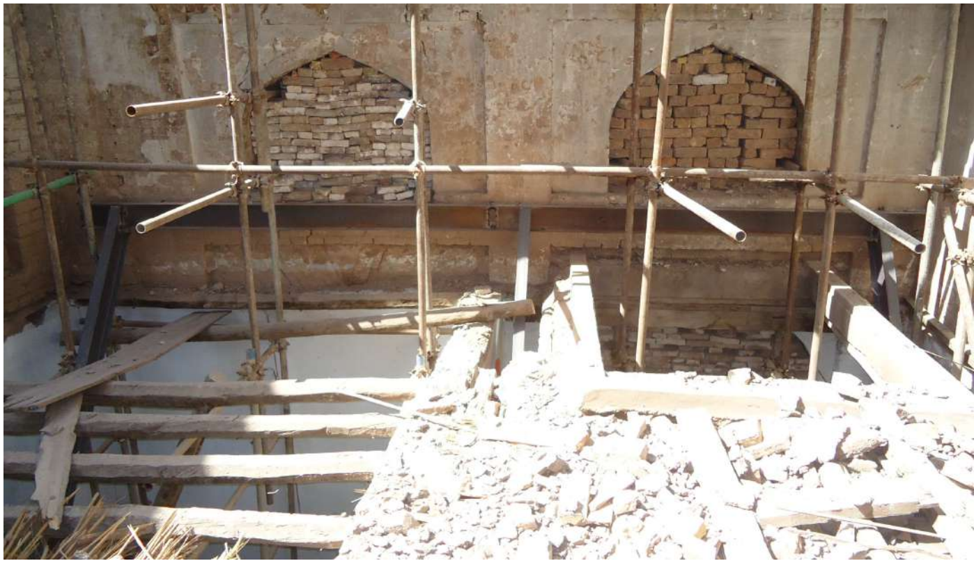
Removal of flooring to reapply water-proofing courses at Level 3,
