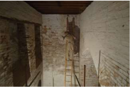
Cleaning masonry.
