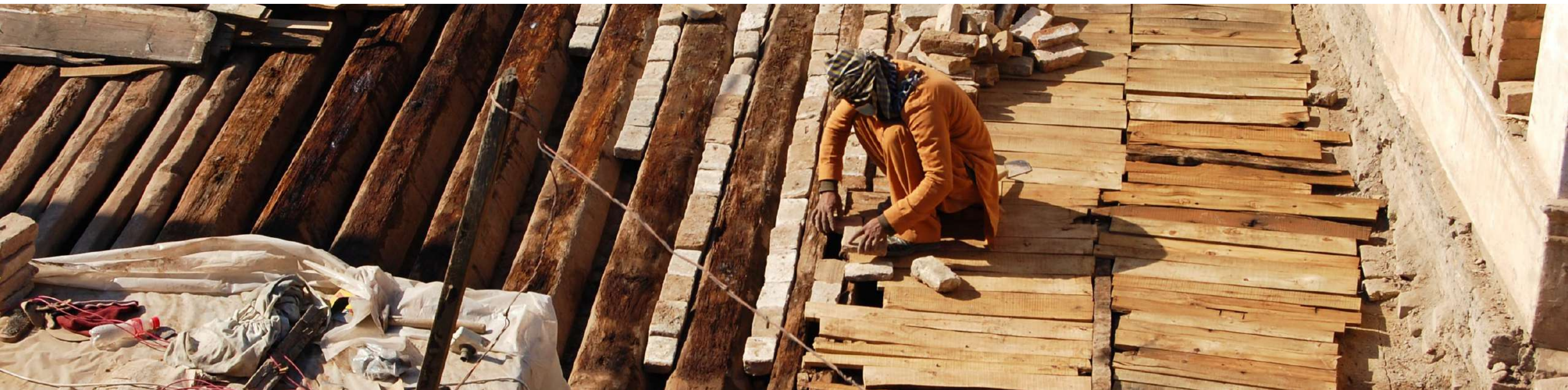
Artisan applies brick and wooden planks to exposed roof.
