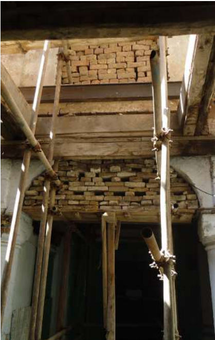
Providing support to Historic section in the rear.
