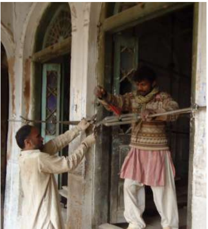
Restraining arrangement of Mid-historic section with cables and clamps.
