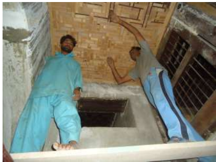
Replacing damaged tarseem bandi.
