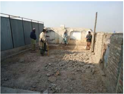
Removal of bricks and compressed earth from roof.
