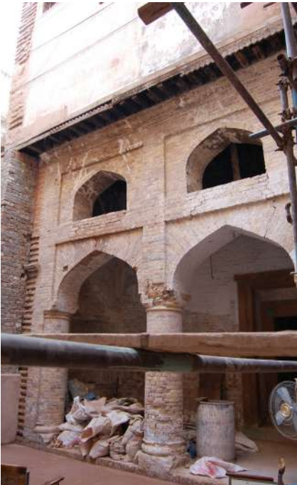
Arches exposed after demolition and removal of later-period brick masonry.
