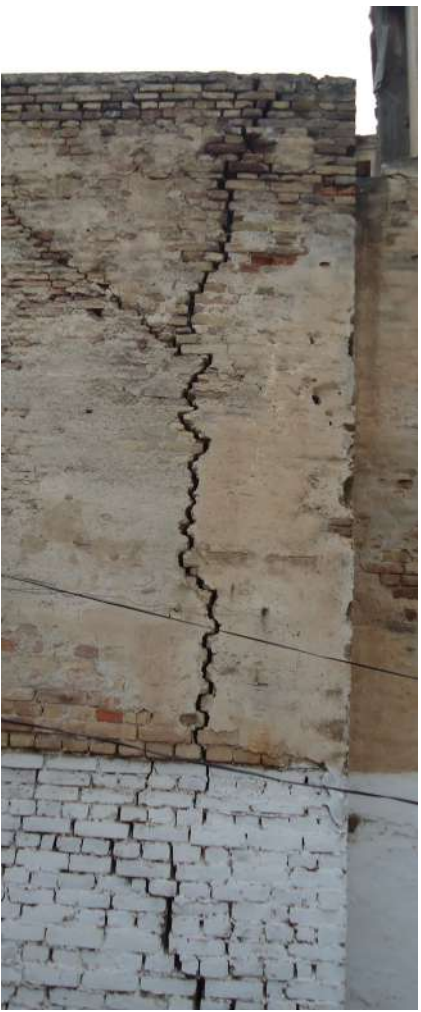
Cracks display structural failure of Mid-historic section.
