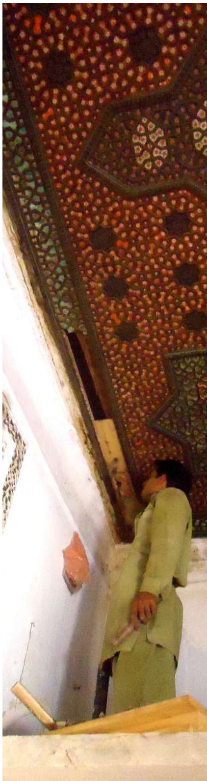
Replacing damaged tarseem bandi .
