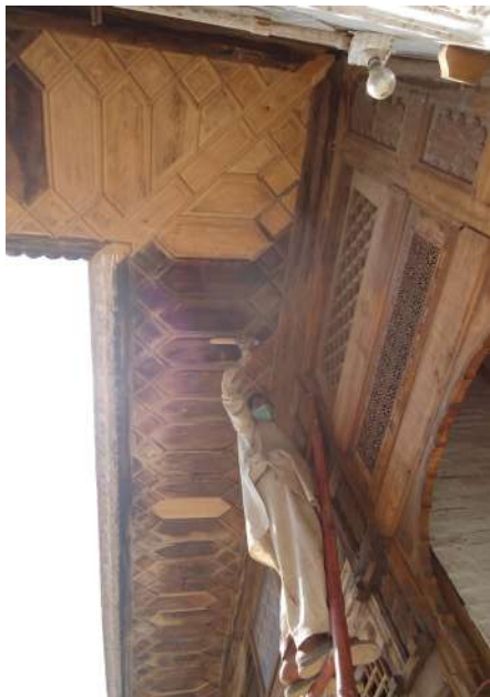
Cleaning tarseem bandi on sun projection.
