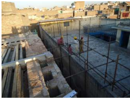
Workers erect scaffolding to begin restoration work on external walls.
