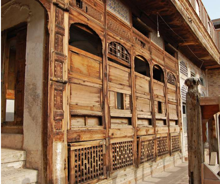
Basta windows on level 3 after cleaning.
