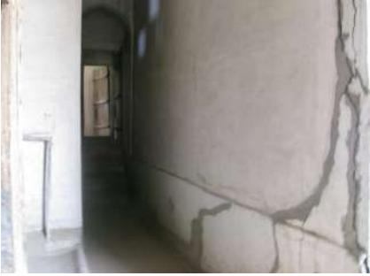
Cracks showing structural failure in Mid-historic section
