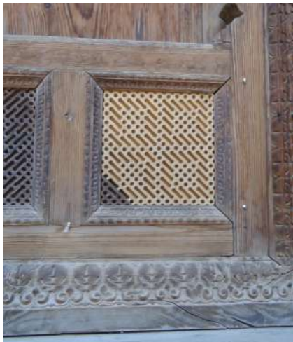
Replacing damaged punjali.
