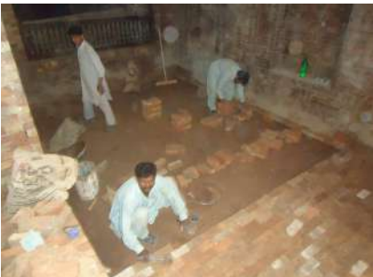
Relaying bricks after filling boreholes.
