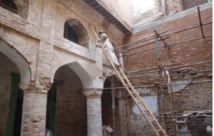
Removal of bricks to expose original openings.
