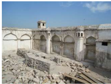
Stacking historic bricks from different locations for reuse.
