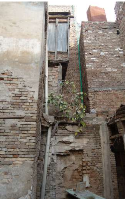
Rear Non-historic section showing damaged brick masonry.
