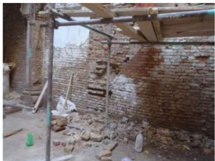
Installing salvaged posts for internal purdah wall.
