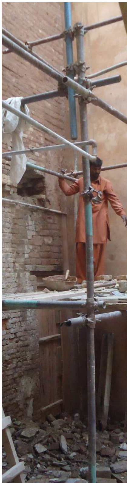
Scaffolding erected so artisans can remove prior interventions and expose original openings.
