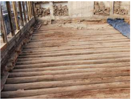
Exposed deodar beams.
