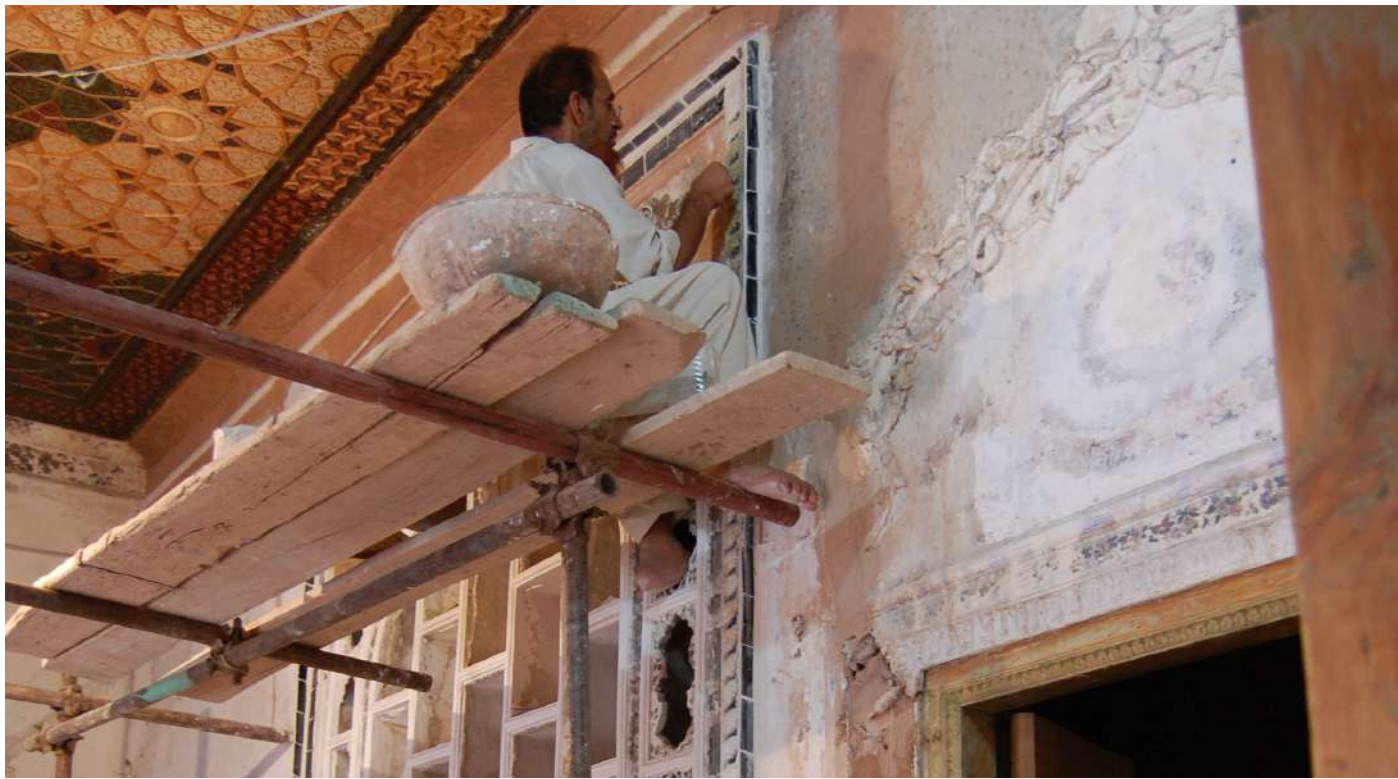
Master artisan prepares stucco tracery around chini kbana.
