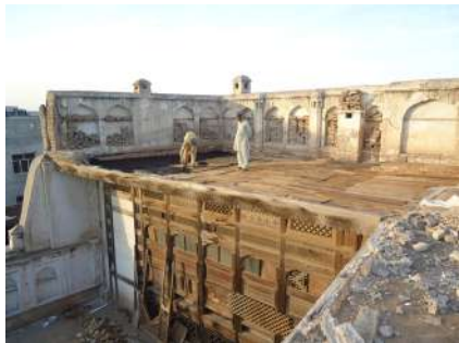
Workers applying anti termite layer on newly fixed planks.
