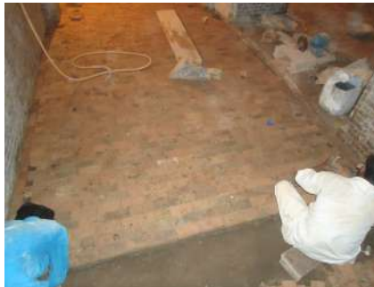
Laying salvaged historic brick after cleaning and new waterproofing in Basement.
