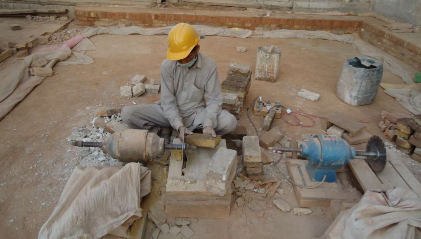
Salvaged brick being trimmed before reuse.
