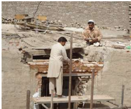
Workers replace masonry and fill cracks in damaged Mid-historic section.
