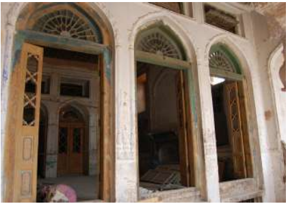
Entrance doors of Room 3/13 during paint removal.
