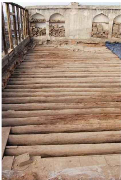
Exposed wooden logs in Roof 4/02 before termite treatment and application of waterproofing and finishing.
