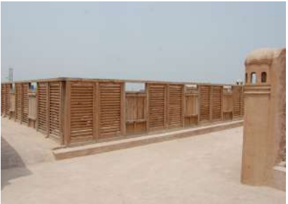
Re-erected and restored wooden Purdah wall on Level 4 Roof.
