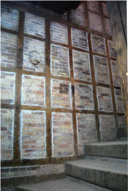
Wood Frame with brick infill walls provide resilience in case of earthquake.
