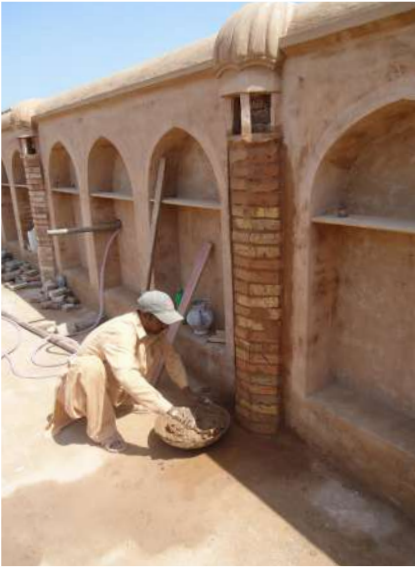
Artisan finishes matching purdah wall with stucco.
