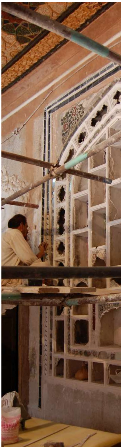
Cleaning and repair of Chini Khana in Room 2/04.
