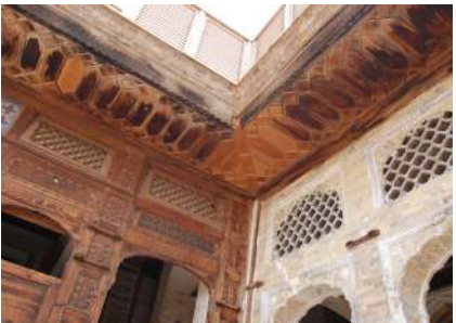
View showing restored tarseem bandi on the soffit of sun projection at Level 3.
