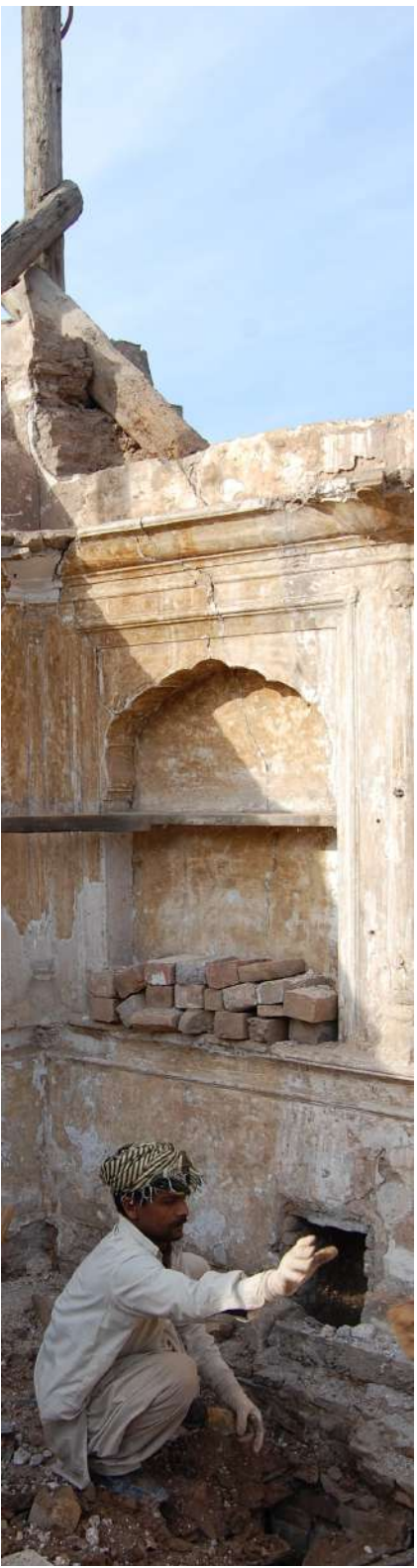
Replacement of Brick Masonry.
