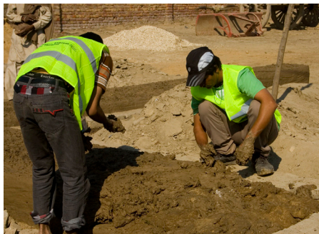
Participants carrying out layered mud construction
