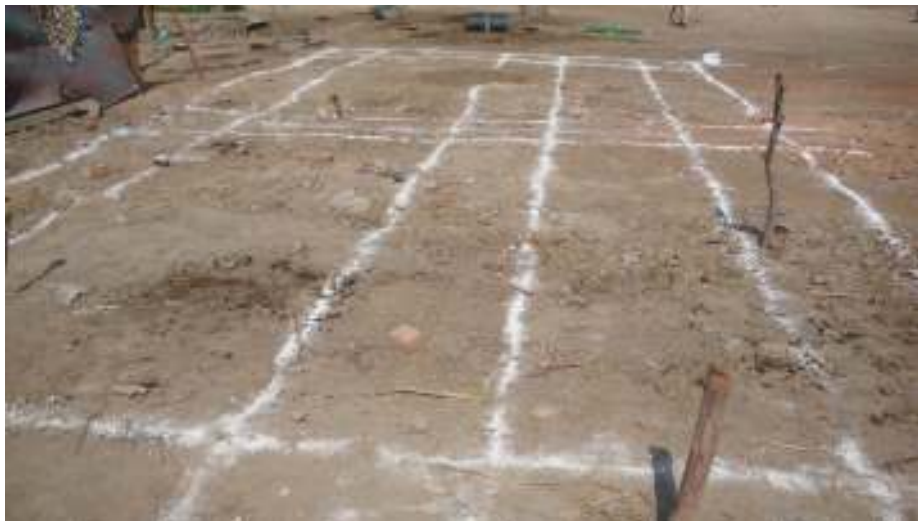
Layout marked ready for household member to excavate GKG foundations
