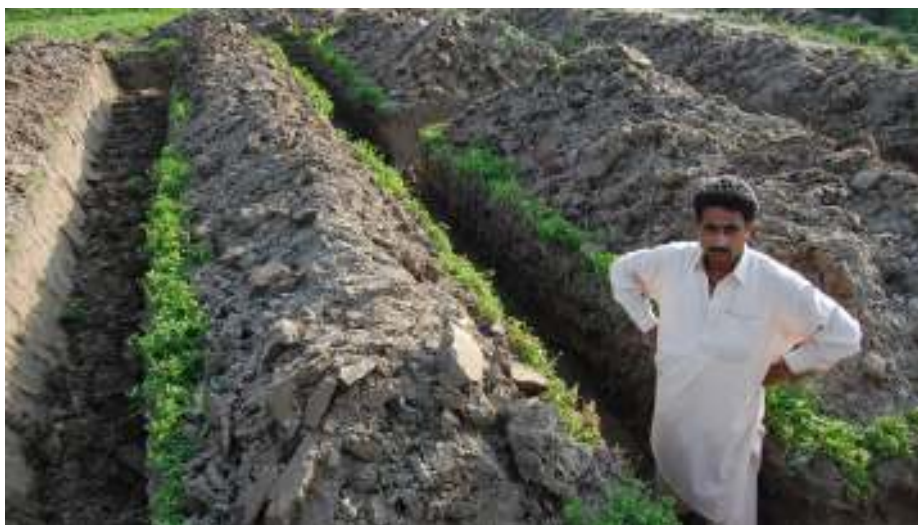
Household member after excavation of GKG foundations
