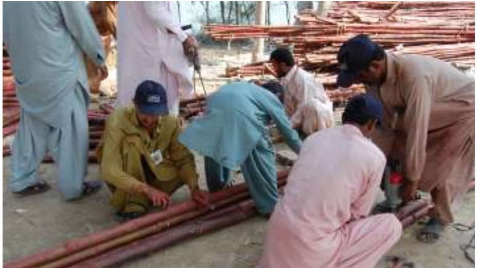
Artisan Trainees learn prefabrication of bamboo joists
