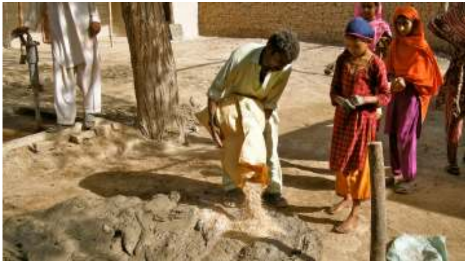
Community members add straw, lime and other key ingredients to make unique plaster
