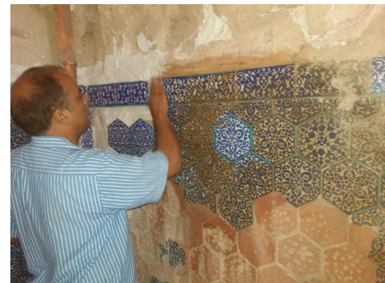
Glazed tile replicas being checked for size and pattern on interior panels carrying hexagonal vegetal interlacement.
