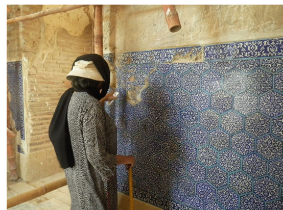
Checking for matching and compatibility of glazed tiles with extant original tiles.
