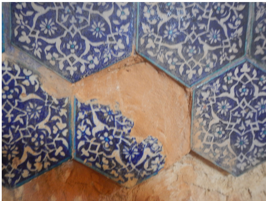
Saving all evidence of original extant kashi, even when in a damaged condition.
