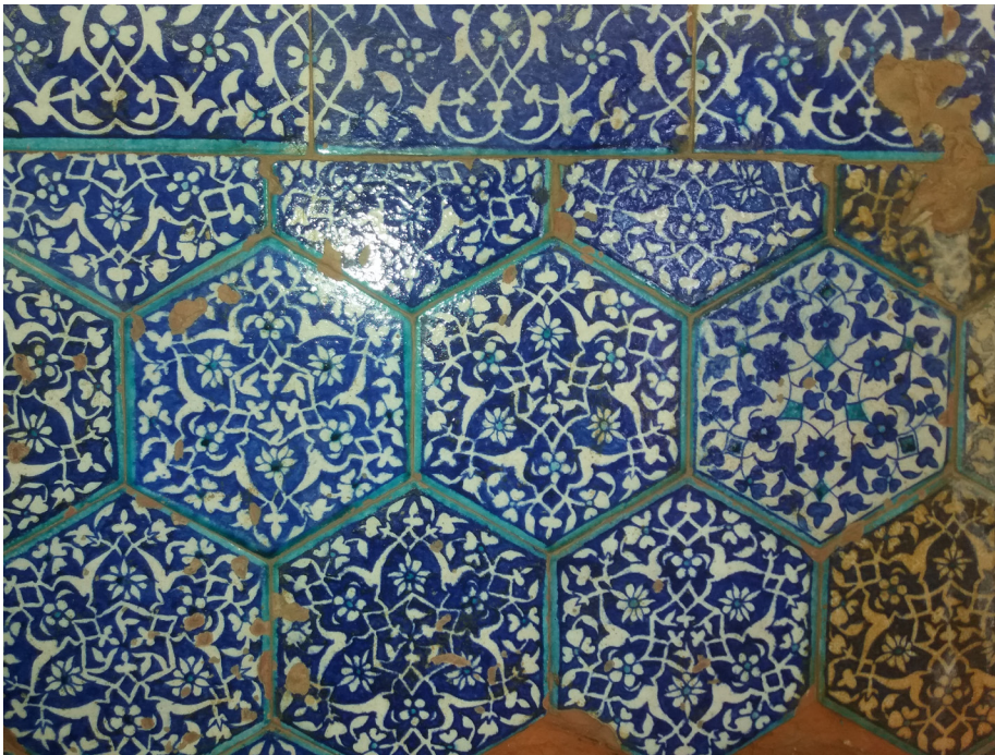
Cleaning and consolidation of original glazed tiles..
