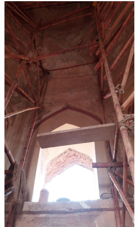
Repairs to window soffits.
