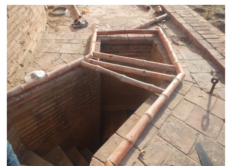
Bamboo roof and trapdoor under construction to prevent water seepage in the stairwell.
