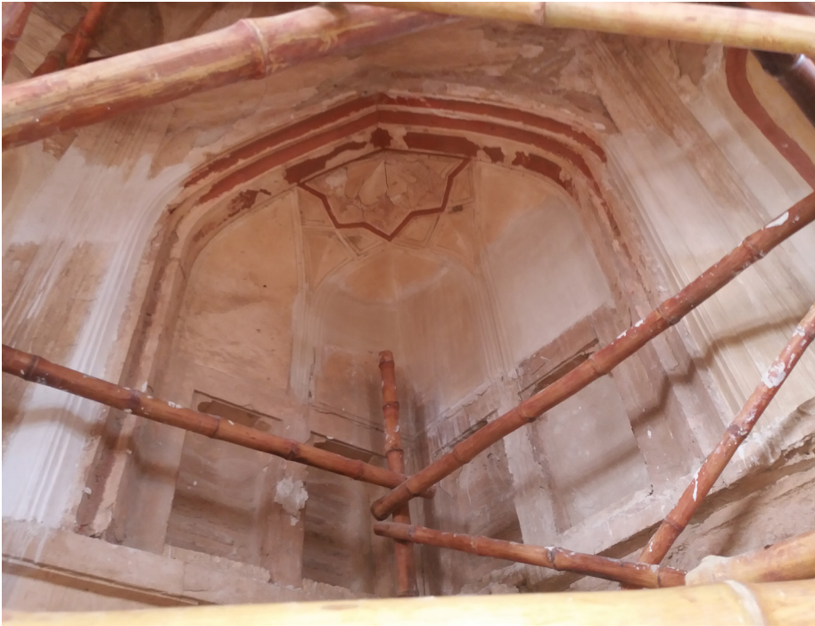
Work in progress on restoration of stucco layers in internal squinch alcoves.
