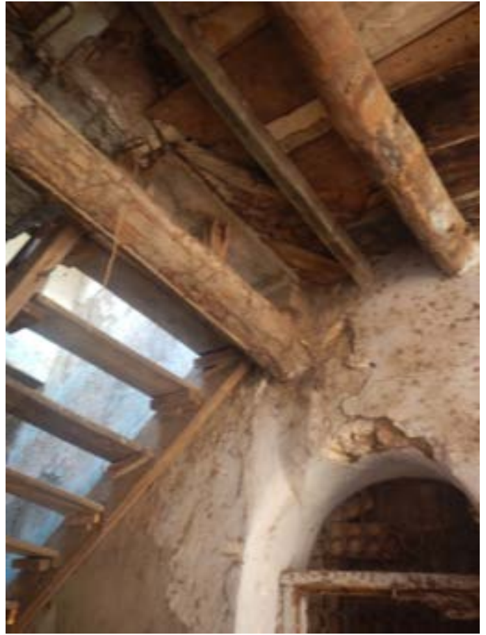
Timber beams at Stair well
