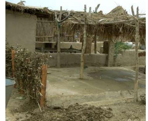
*The enclosure can also be covered with a low cost reed roof.*
