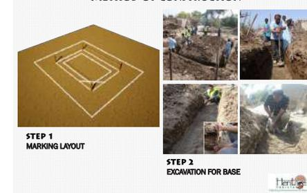
Mark the layout, Internal Edge of Wall: 3'-6" x 5'-6", External Edge for Toe: 9'-3" x 11'-3". Remove top soil & excavate 1'-6" below ground.
