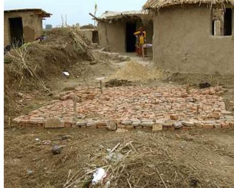
*Hard core provides strength for flooring.*
