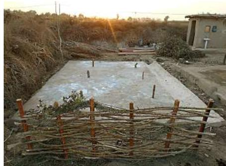
*The low-cost Majandri tree fence allows for air to cross through.*
