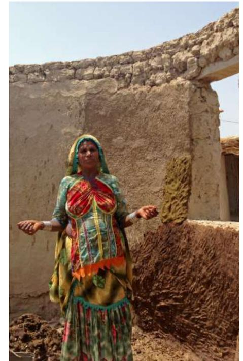
*Application of lime/mud/sand plaster mixed with chopped straw and dung.*
