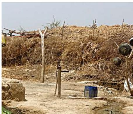
*Common hand pumps are subject to contamination by being so close to the ground.*
