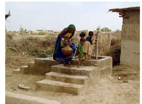
*The raised platform helps keep the hand pump area and water source clean.*
