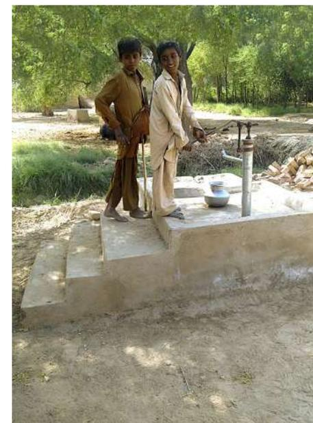
*The raised platform and use of lime make the hand pump DRR compliant.*
