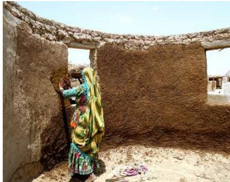
*Construction of mud walls and application of first layer of mud plaster.*
