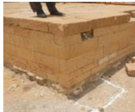
Exposed plinth stone of Entrance platform.
