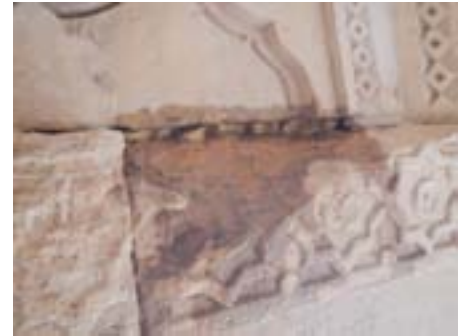
First layer of injected mortar
