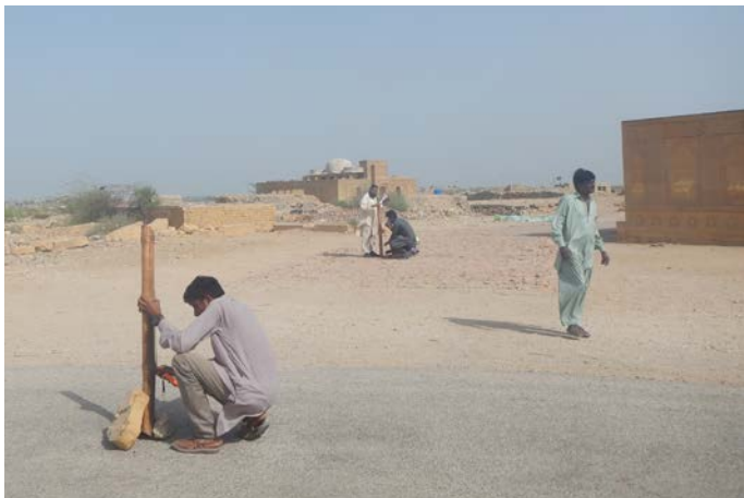
Checking the building levels in reference with the road.
