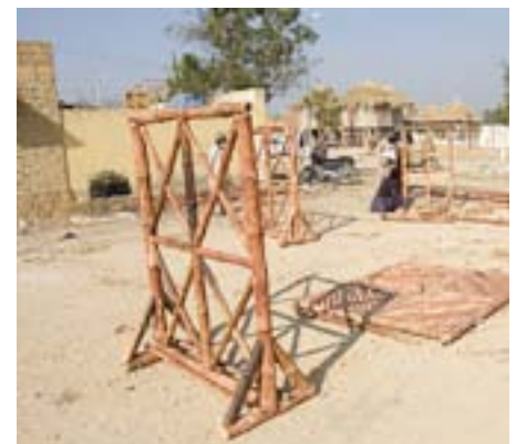
Fabrication of free standing bamboo barriers
