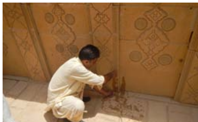
Checking the floor levels with a water-level
