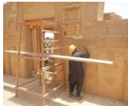
Artisan, dry clean the walls of the enclosure
