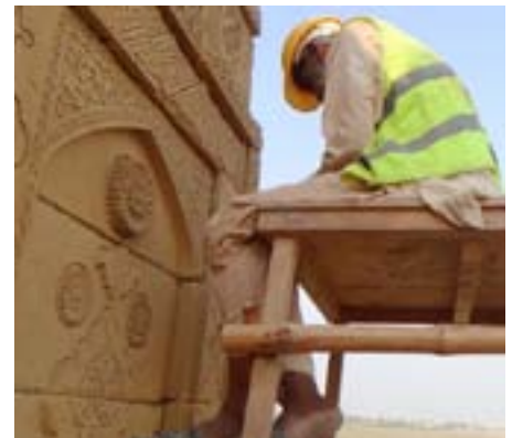
Pointing on the exterior facade of the Tomb.
