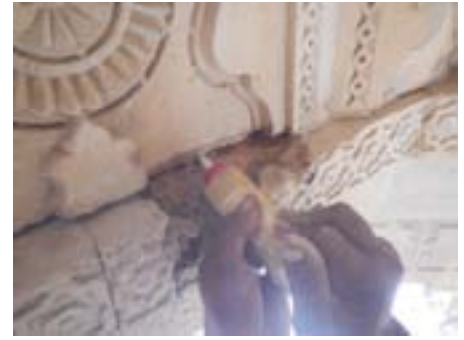
Injecting Lime Mortar into deep joints
