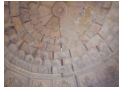
North East Section after Brick underpinning
