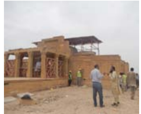
Tomb of Jan Baba with bamboo barriers and temporary roof providing protection.
