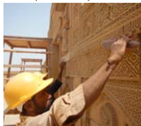
Dry cleaning through careful light brushing
