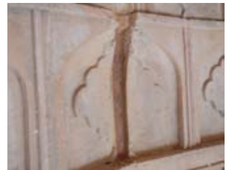
Close-up of the terracotta piece profiled to fit in the gap.
