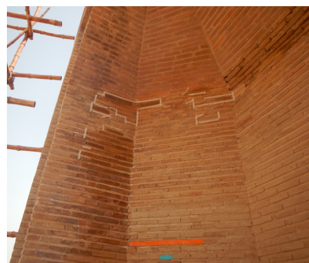
Areas treated by underpinning
