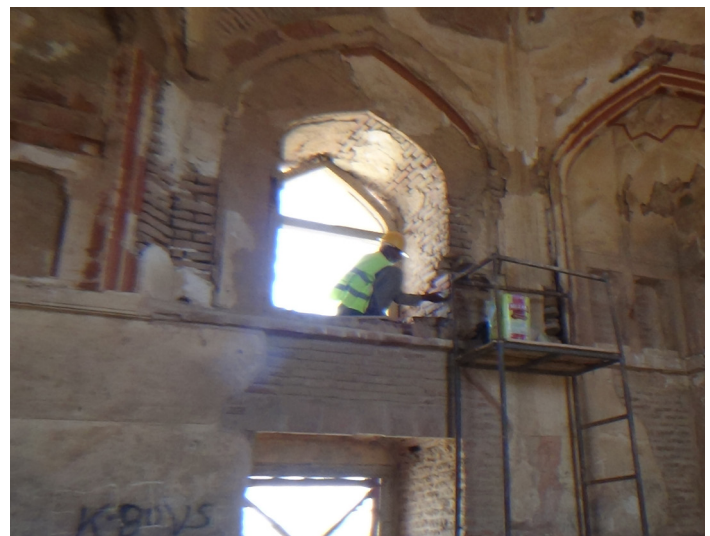
Pointing of the interior walls.
