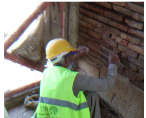
Pointing of mortar joints.
