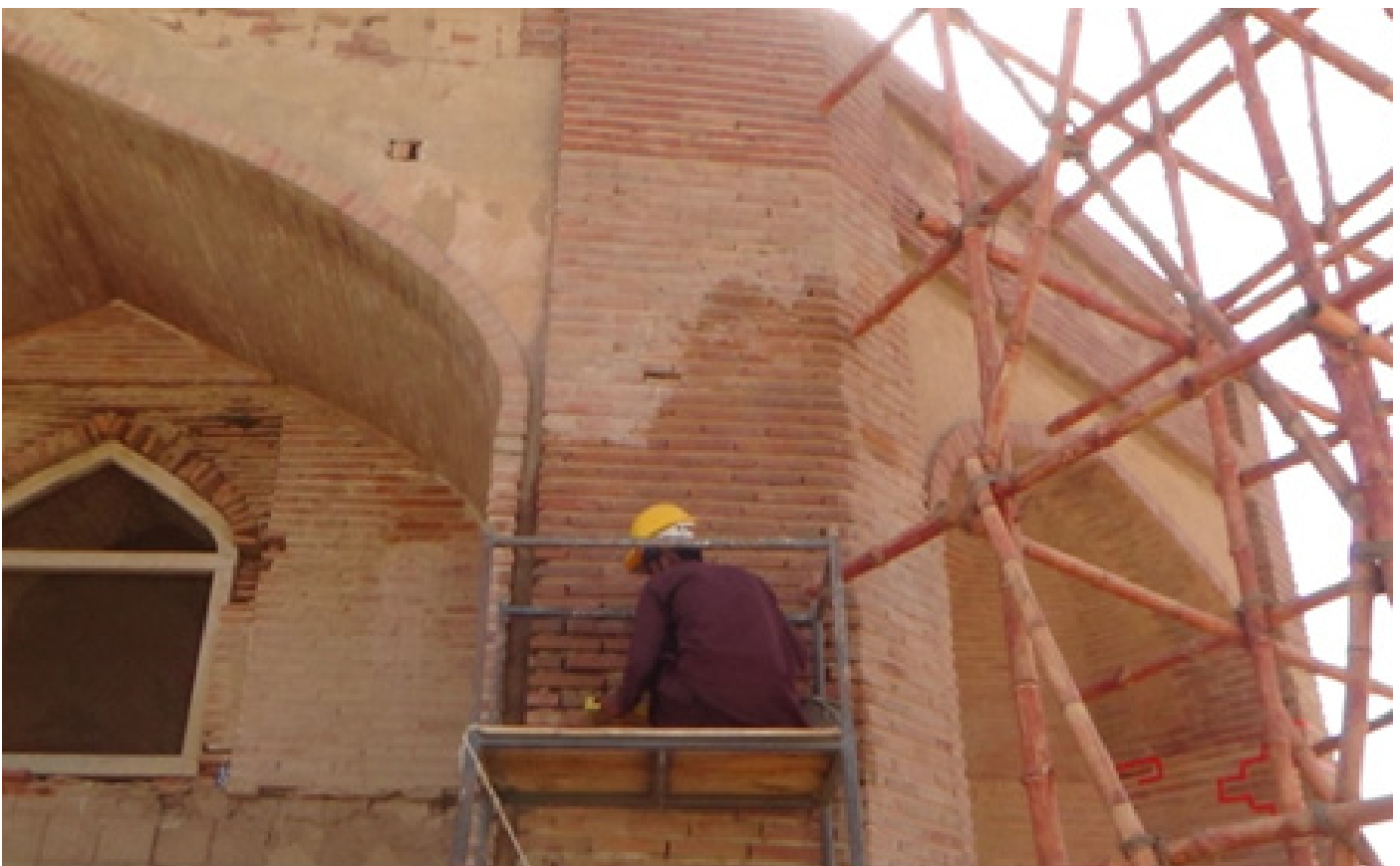
Artisans treating the mortar joints by pointing
