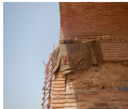
Curing of mortar joints
