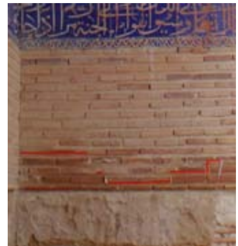
After the completion of underpinning.
