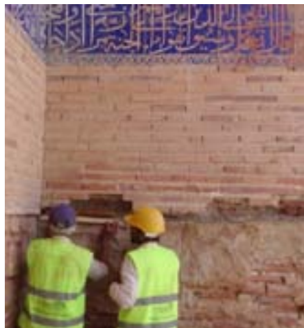
During the underpinning process.
