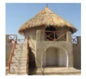
Built with the help of Murad Jamil, the Jamil ParhoPakistan Centre utilizes mud brick vault on ground floor with mud walls supporting a bamboo chaura thatched roof, providing a picturesque view. The construction of mud vault has been successfully carried out, providing providing a channel at ground floor for disposal of flood waters, and a cool shaded place for children's activity during normal conditions. The design employs traditional way of building arcuate strctures common in the region.
