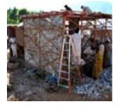
The bamboo dhijji (cross bracing) has been utilized in housing units built in Swat. Since its construction many seismic jolts have been experienced which the housing units have withstood. The dhijii allows the use of local materials as filling between the cross bracing which is an economical method of construction. The structure is strong enough to withstand earthquake as well as floods. Training provided to communities allows them to self build structure themselves.
