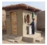
This is the protoype of eco-toilet that was first built to try out the possibilty of acceptance of such toilets. The mud walls and KaravanJoist roofs also provide possibilty of roof farming or Chhat Bagheecha. The two-seat box provides separation of liquids (drained into a plantation bed) and solids (collected in a bucket). The solid (night soil) is removed to a composting bin which is maintained by a Khad Adhi (Compost Sister) who purchased the night soil to make compost.
