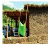
The first protoype of a house using bamboo dhijii cross bracing and bamboo joists in roof that waa constructed.in Swat and soon after over three hundred housing units were built in the difficult to access hilly terrain of the area. The housing units were supported by the University of Glasgow & Scottish Government International Development Fund (SGIDF). Although the technique was entirely new, but it was readily embraced by the communities due to its insulation value in the cold climate of Swat.
