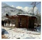
Based on the bamboo cross bracing developed for the Zero Carbon Footprint house in Swat, a Green Women's Centre was built in village Beha in Matta in an area that had been wrecked by militants. This was the first bamboo roof with a span of 16' and it was tested the same year when the snow piled up 3' to 4'. This was also the first centre that was built for women. Later a few more centres were built by the Foundation in order to provide socializing and working space for women in Swat.
