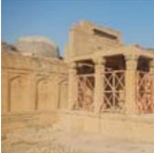
The stone tomb of Jan Baba, originally an enclosure, that later seems to have acquired entrance and grave canopies along with separation of a zenana enclosure. The graves canopy has suffered due to the settlement in the middle chamber and loss of two valuable domes. The effort is to maintain the original stone work as well as preventing the collapse of the middle dome fabricated with neatly arranged carved stone tiles. The project is supported by the German Government.
