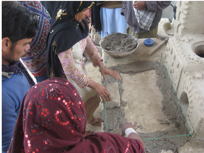
Champa guiding the trainees to build the combustion chambers.
