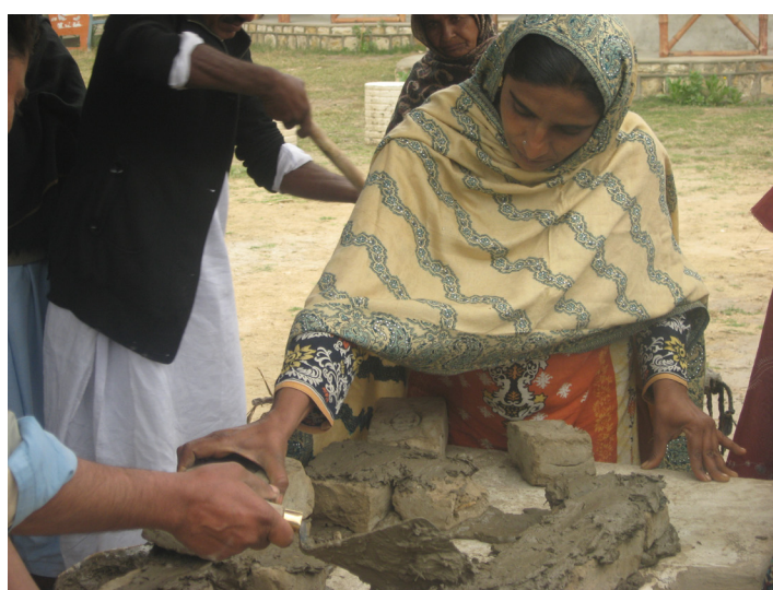
A couple building the mud walls for the stove chambers.
