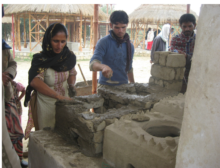
Another team working on the mud walls for the stove chambers.
