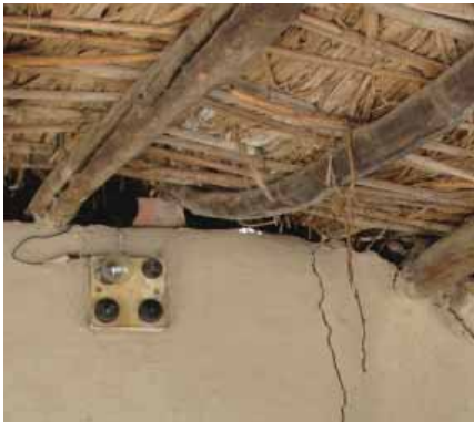
Local soft wood joists prone to termite damage, and unable to carry extra load.
