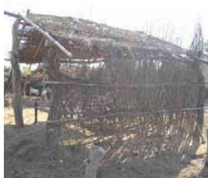
Badly constructed Loh-Khat walls suffer damage
