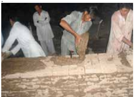
Sun-dried brick wall construction.
