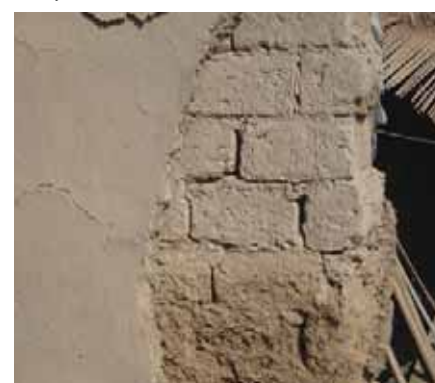
Damaged wall that is structurally stable and can be rehabilitated.
