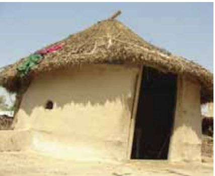
Conical roof structure with well plastered reed walls.
