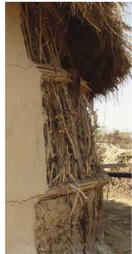
Reed wall construction. Eroded mud plaster render and lack of protection at the base.
