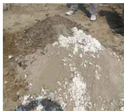
Mixture of lime, mud and bhoosa (straw)
