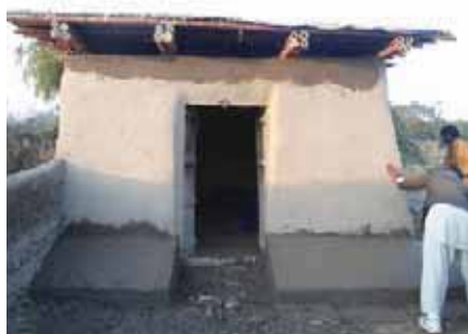
A model/demo unit with mud walls, mud toe base and KaravanRoof.
