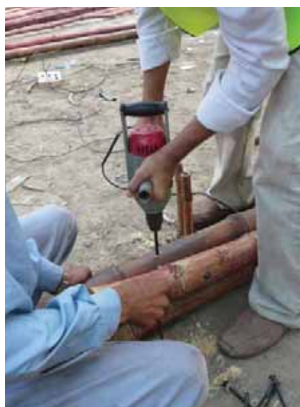
Using an electric drill to bore holes for jointing bamboo
