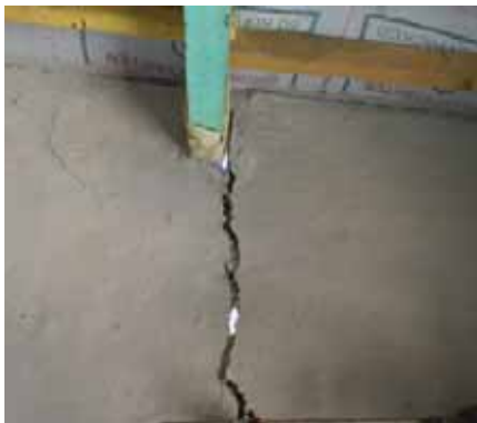
Above. Major crack in the supporting mud wall due to the point load of a steel girder.
