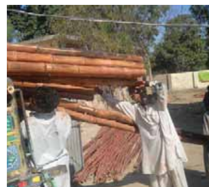
Prefabricated bamboo joists being transported to other locations for use in demo/model units.
