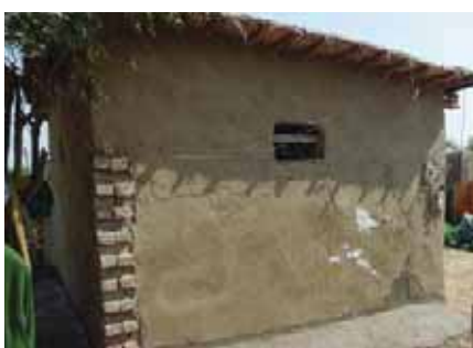
Building a toe for extra support to walls
