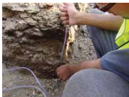
Ensure alignment of wall with a rope at all layers of mud courses
