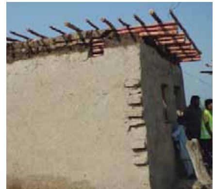
View of another KaravanRoof under construction.
