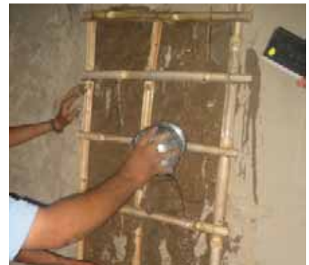
Fixing of bamboo lattice on the damaged area of the wall.
