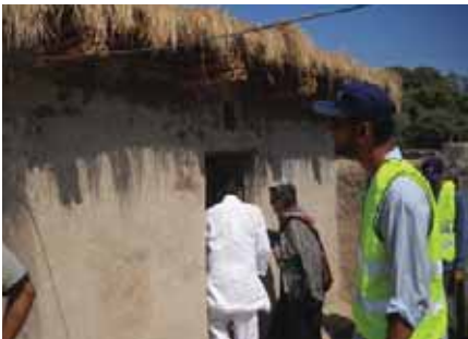
A completed unit with lime-mud rendering.
