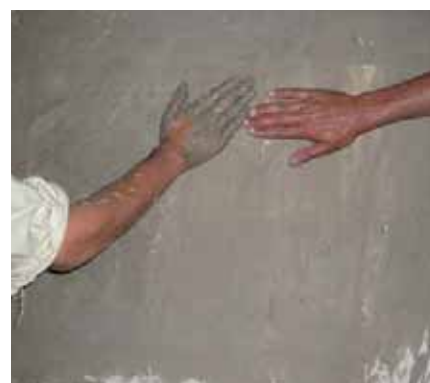
Lime render must be smoothed after application
