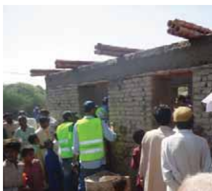
Model shelter constructed with sun-dried brick and KaravanRoof.
