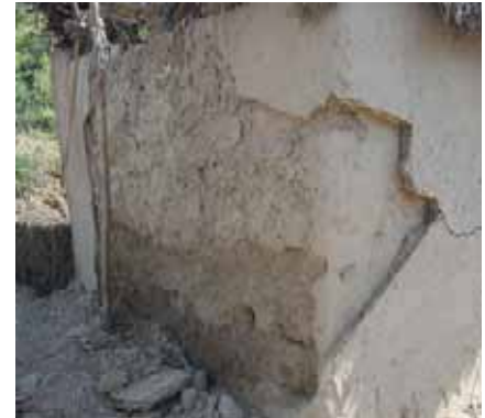
Heavily eroded base of a mud wall, making the structure vulnerable.
