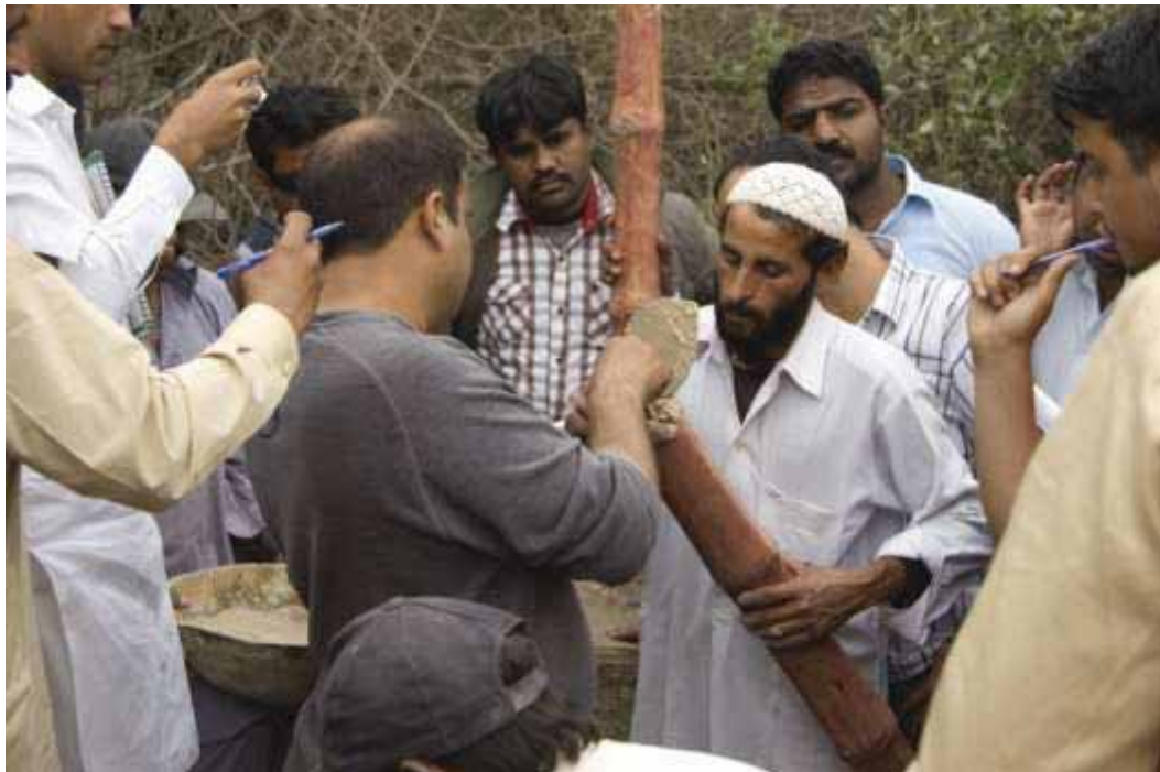
HF team demonstrates method to grout steel bar in bamboo post
