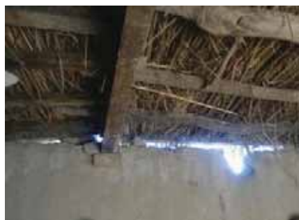
Damage to walls due to lack of lintol
