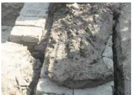
Laying mud brick in mud mortar in plinth.
