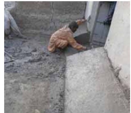
Extra plinth in the form of a toe to provide protection to the base of a mud wall.
