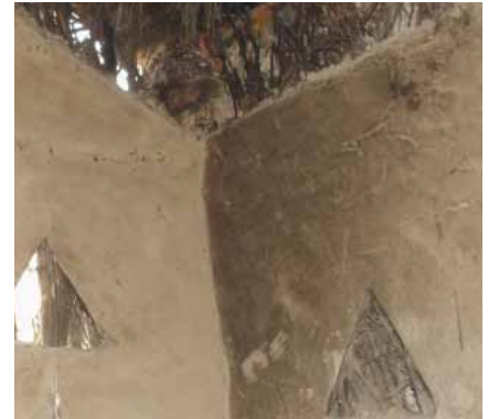
Seepage of water through badly constructed roof making the structure vulnerable.
