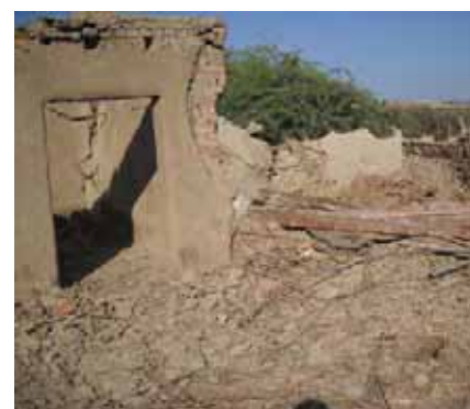
Collapsed roof due to poor construction
