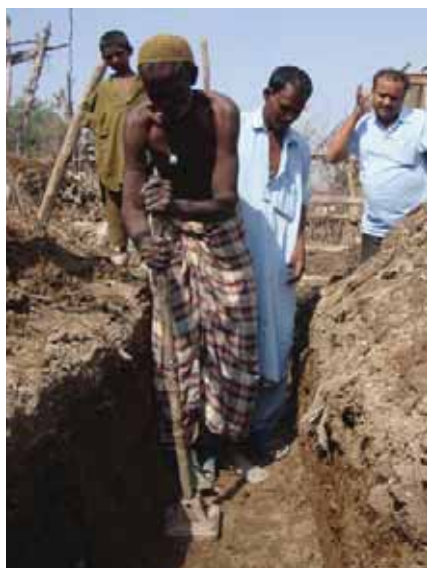
Tamp earth to ensure firm footing
