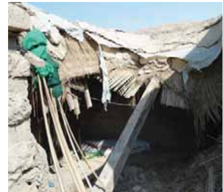
Extra dead weight on a roof causes the collapse of the entire structure.
