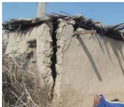
Incorrect construction techniques lead to cracks in walls.
