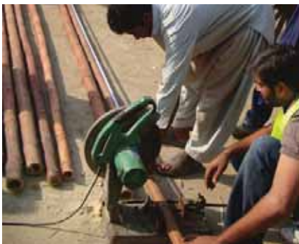
Prefabrication of bamboo joists in progress..
