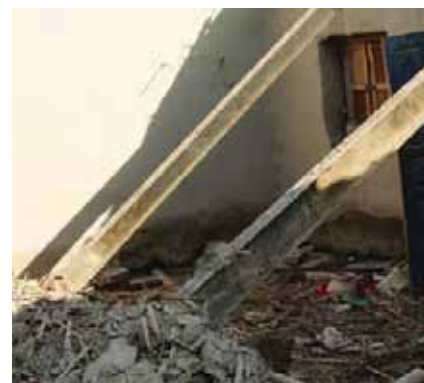
Collapsed wall and roof due to use of heavy steel girders.
