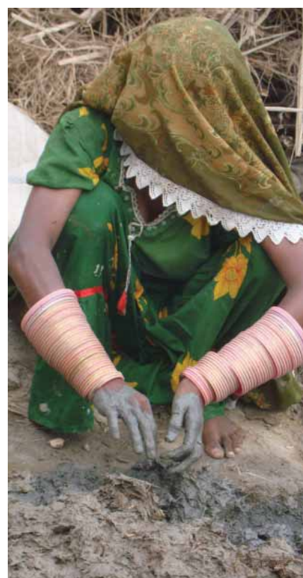
Making mud-lime mix for wall rendering, allows participation of women in rehabilitation of their houses.
