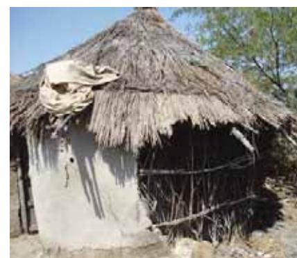
Conical Chaura construction with disintegrated plaster
