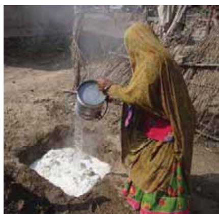
Mixing lime for slaking
