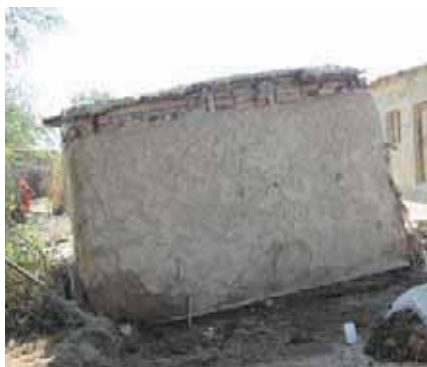
Structure displaced due to a highly damaged base.
