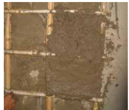
Mud plaster being applied over bamboo lattice, thus saving a damaged wall.
