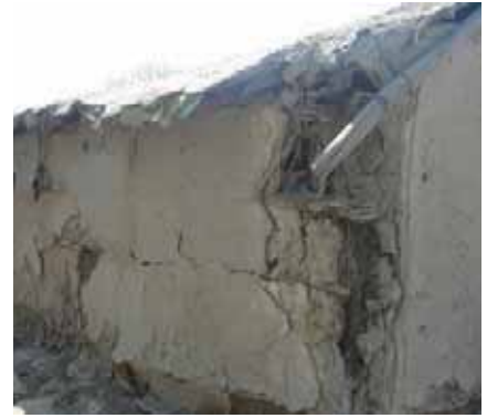
Vernacular construction damaged by standing water.
