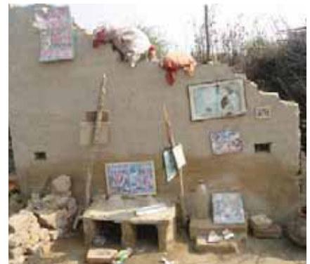
Partially collapsed mud structure selected by Heritage Foundation for rehabilitation.
