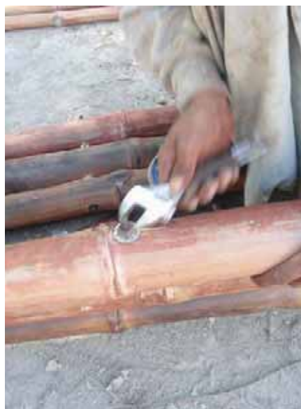
Tighten and secure nut and bolt
