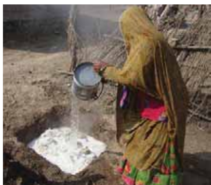
Woman participating in the construction process - mixing lime in a lime pit.
