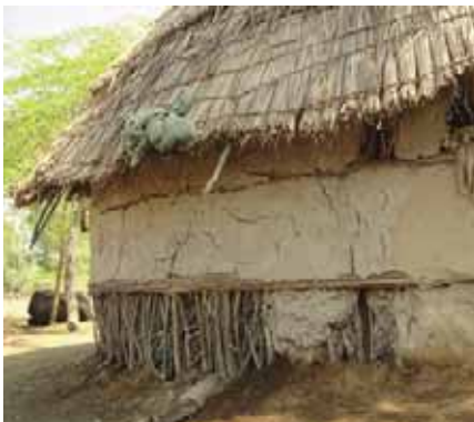
Disintegration of mud plaster on walls. The base is entirely vulnerable.
