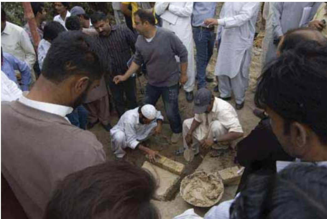
HF artisans demonstrate method to make pad at base for bamboo posts
