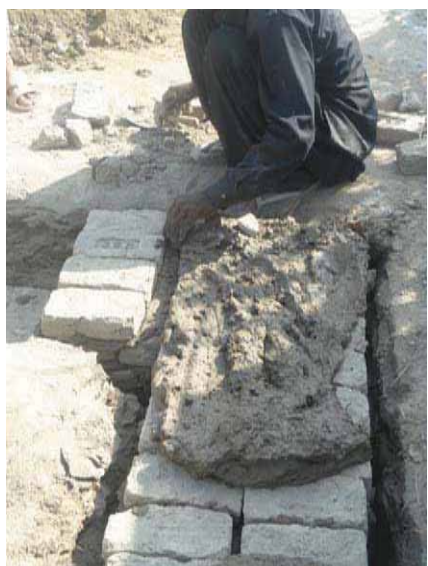
Mud walls should be at least 18" thick
