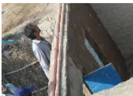
Placing bamboo reinforced lime concrete ring beam to receive bamboo joists.
