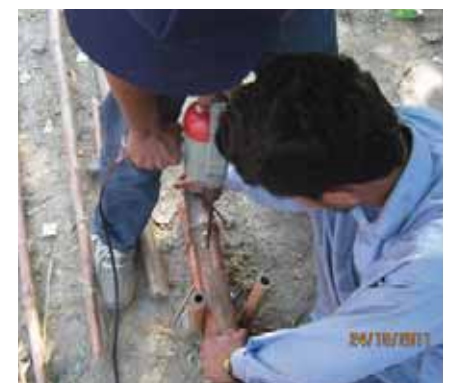
Trained HF artisans demonstrating fabrication of bamboo elements.
