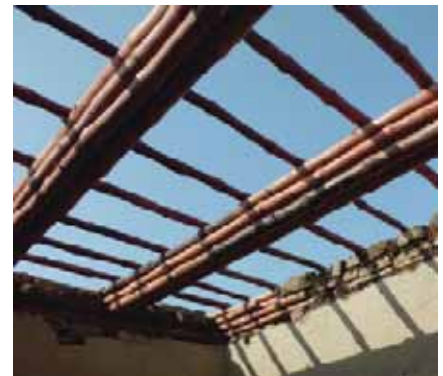
View of safe-haven KaravanRoof being installed.
