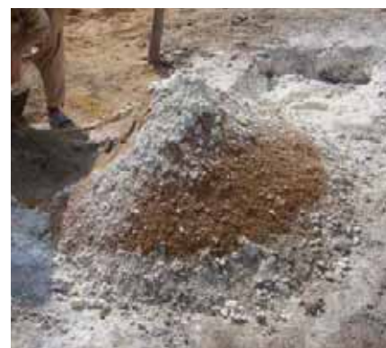
Mixing lime with soil to prepare mortar
