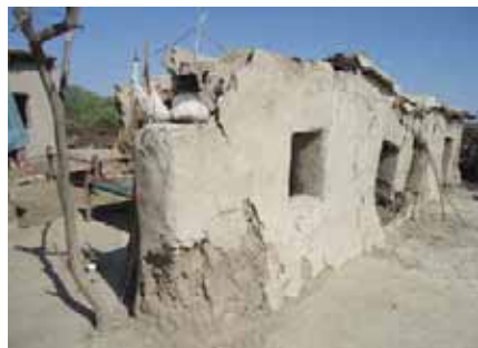
Damage to unit due to lack of ring beam
