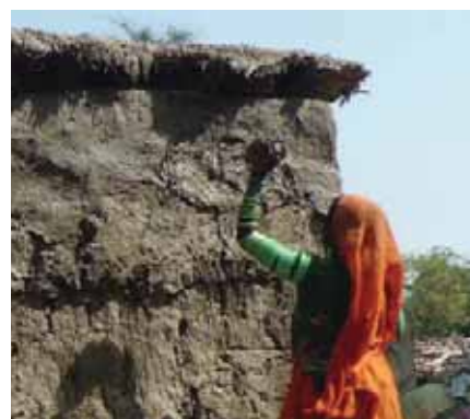
Lime render to be applied by hand
