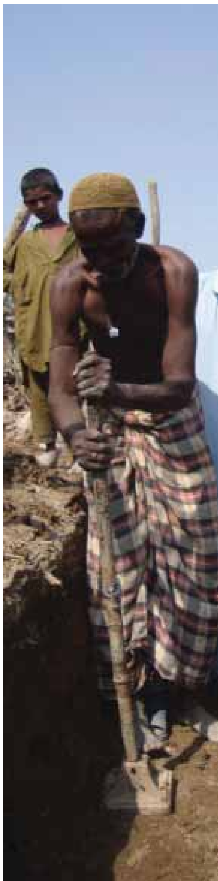
Local community participating in rehabilitation, tamping the soil well to create a firm base.
