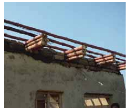
Placement of bamboo purlins on bamboo joists.
