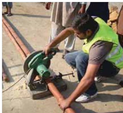
Cutting bamboo with electric saw
