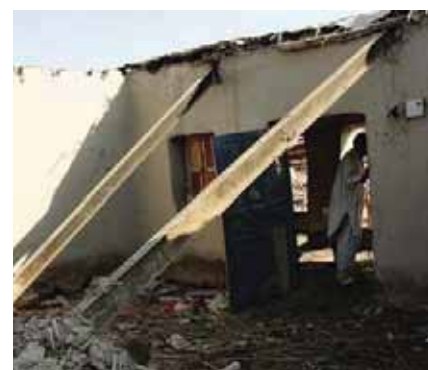
Collapsed steel girders.
