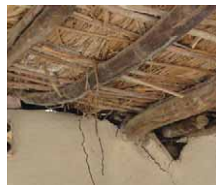
Heavy logs and bamboo used for roof construction damage walls
