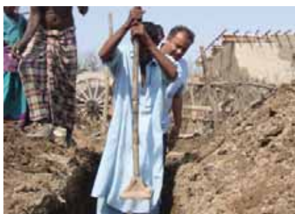
Excavation & tamping for firm ground.
