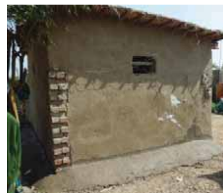
DRR-compliant rehabilitated unit with lime rendering, ground toe and Karavan-Roof.
