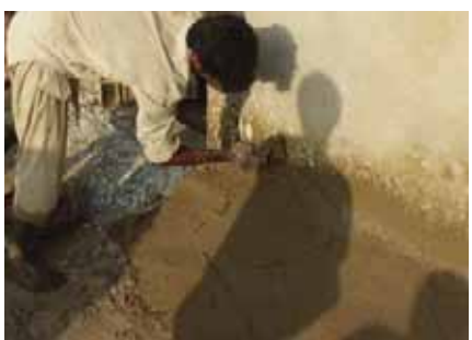
Making a mud toe at base of mud wall.
