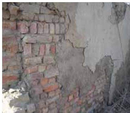
Fired brick walls built without proper bonding or mortar
