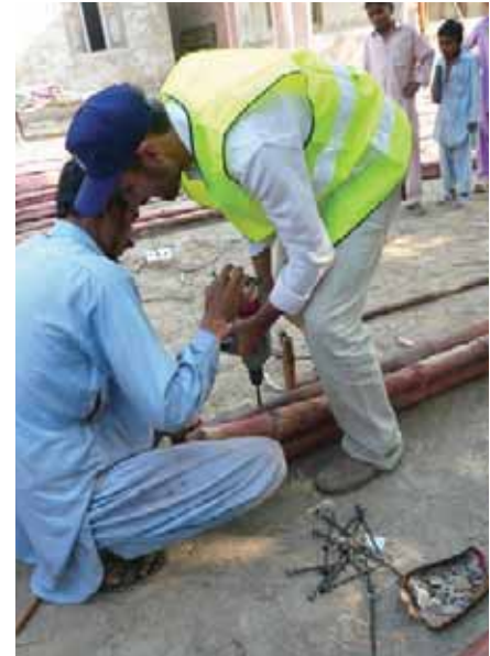
Artisans being trained in prefabricated bamboo joist production.
