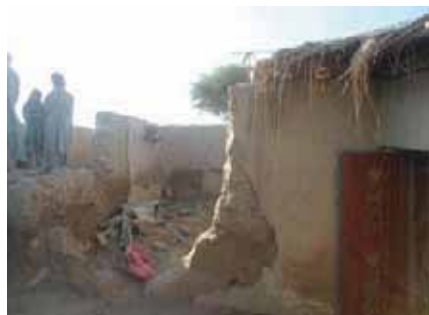
Damage to walls due to lack of plinth
