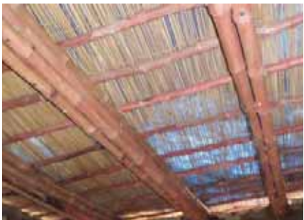
Installation of KaravanRoof in place.
