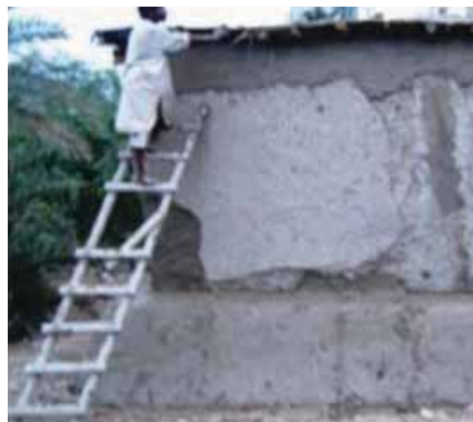
Raised floor from the ground level provides protection from flood waters.
