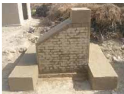
Demo sample, mud brick base with toe for inaccessible roofs
