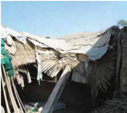
Collapse of ill-built roof structure.
