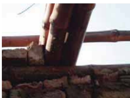
Bamboo joists and ring beam must be tied securely
