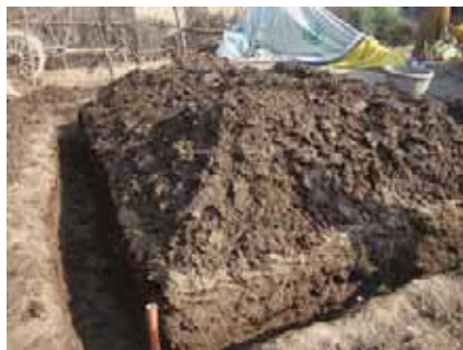
Excavation to 450mm below ground level
