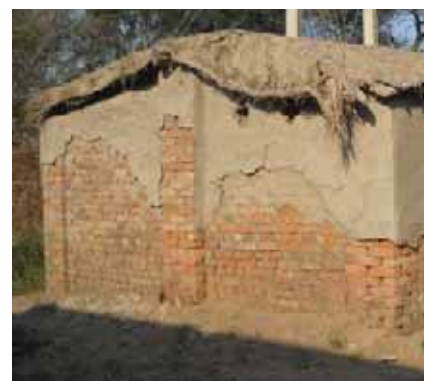
Usual pitched roof construction supported by poorly laid burnt brick walls.
