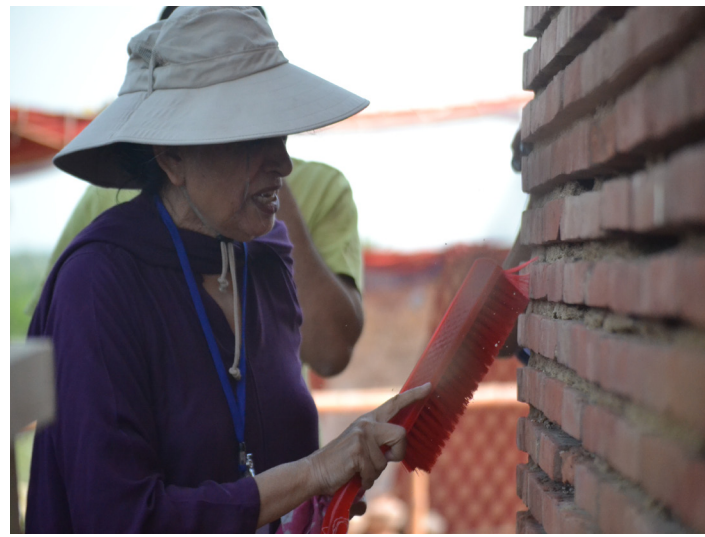
CEO Heritage Foundation Mrs Yasmeen Lari demonstrating dry cleaning of brick walls.
