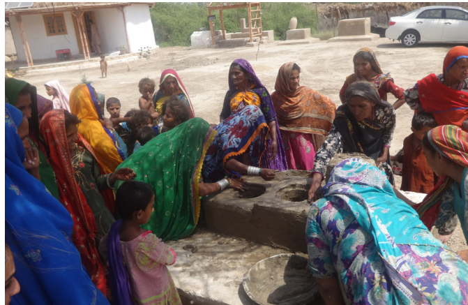
Plaster rendering is an important step to ensure an efficient stove
