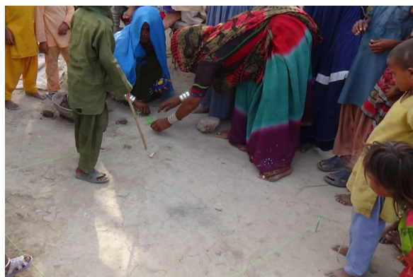
Trainees learning how to mark layout for tiba construction
